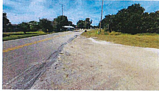
LAKE BRANCH RD FACING NORTH
